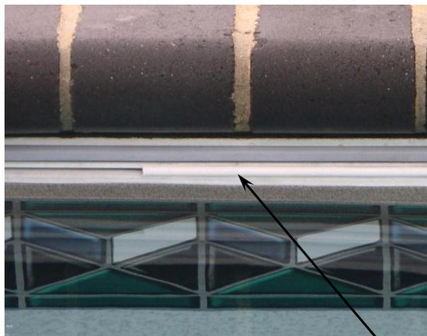
Beadlock installed in a section of tracking
