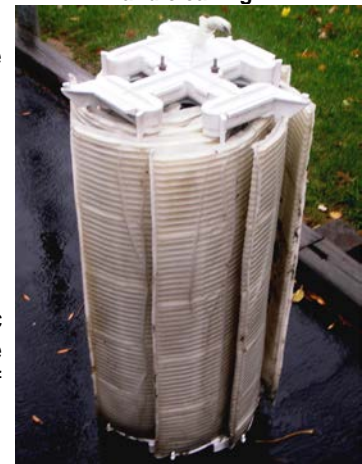
Same filter after dismantling and cleaning
