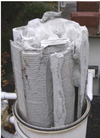
Filter after customer back washing (prior to cleanout)
